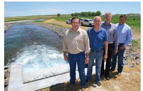
Platte, Neb., in Lincoln County. The property, when purchased by NCORPE, had 115 irrigation wells; now retired, 30 of those wells have been converted to augmentation wells that are tied to a 42” main pipeline that discharges water into Medicine Creek. Like Rock Creek, Medicine Creek is a tributary of the Republican River. At full capacity, NCORPE can annually produce approximately 65,000 acre feet of water and, like Rock Creek, is actively being restored to native rangeland.
